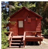
Leydon Cabin – Sleeps 4 (bathroom)
